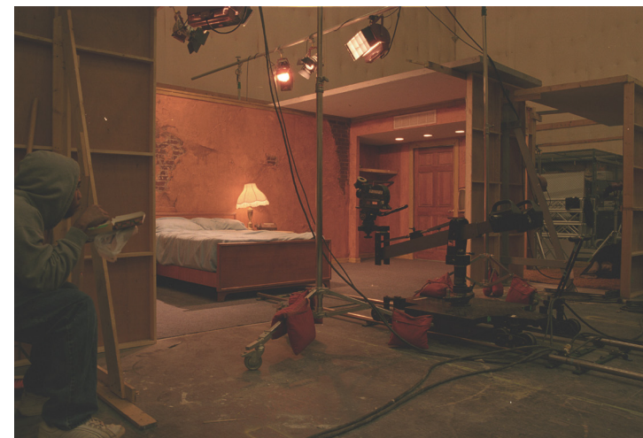
Motel Room: Art Director/ Construction Coordinator. Built on stage, this 360 set had several fly-walls for flexible shooting and lighting.
