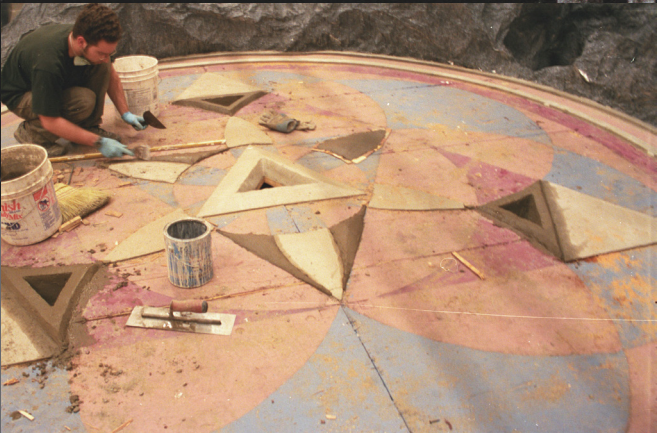
Mountain Top/ Ceremonial Platform: This set is 30 feet in diameter built on top of a 4 foot steel platform. The background was simply blacked out for digital replacements. The Platform finish was created from individually sculpted concrete panels.
